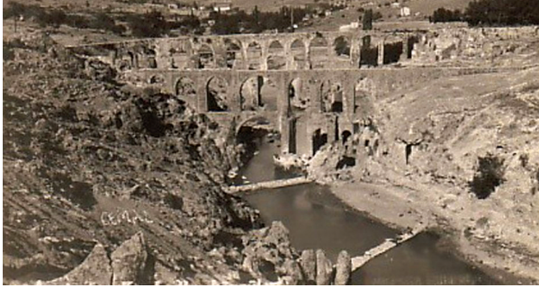
The Kızılçullu Aqueducts that were used to carry the water that gave life to İzmir.
