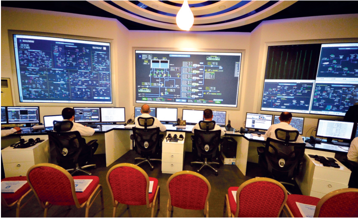
SCADA forms the backbone of İZSU's potable water distribution system.
