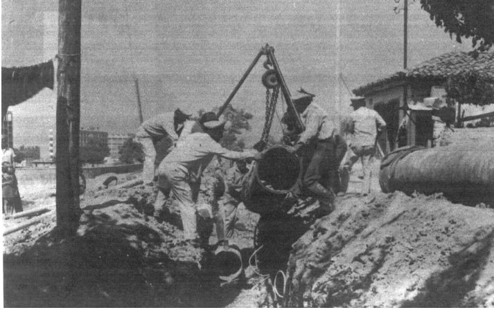
A view of the 500 mm distribution line furbishing between the Halkapınar Water Factory and the Kadifekale Water Tank.
