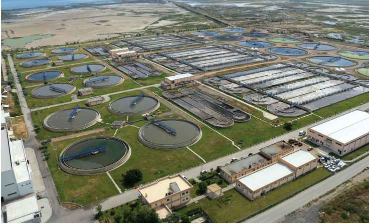
Çiğli Wastewater Treatment Plant has Turkey's biggest advanced biologic process with its capacity.
