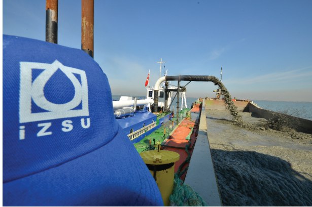
A view from dredging operations in the İzmir Gulf.
