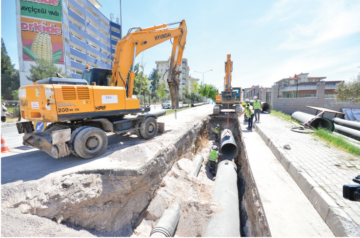
A view from the constructions of the transmission line that will be carrying water from Gördes Dam to İzmir.
